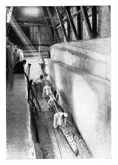
B.—Tying the piece with ropes hanging down from the iron beam.
