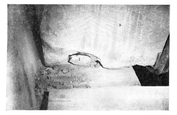
A.—Part of the north west corner of one of the blocks showing: (1) The northern semi-circular opening filled with gypsum mortar. (2) The trickling down of the thin gypsum mortar which was poured from above to fill the small spaces between every two adjacent blocks.
