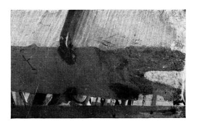
B.—The semi-ellipsoidal opening in the extremity of the bottom surface of a block.
