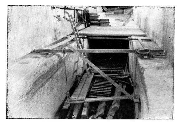
B.—The beams, boards and ropes composing the scaffold and the way they were put together.
