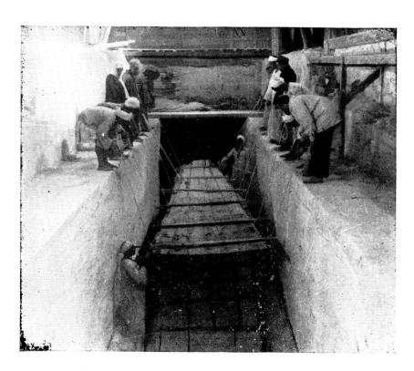
A.-Repeating the unit of the scaffold and tying the cross-beams with ropes.
