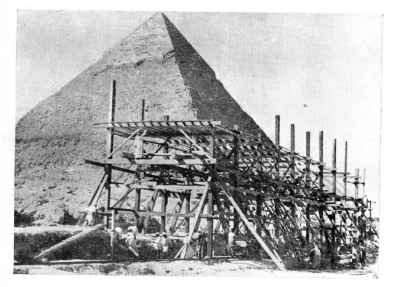
$B_{\bullet}$ —Erecting the skeleton of the shelter.
