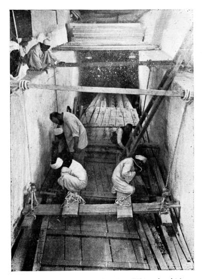
A.—Putting the longitudinal boards of the scaffold inwards and tying the cross-beams with ropes.
