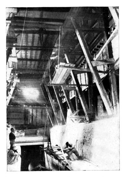
A.—The crane hung in the roof of the shelter. An iron beam tied to its hook and hanging in the pit.
