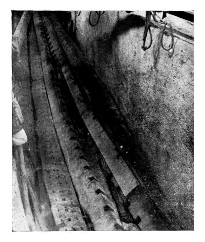
$B.-\!\!-\!\!\operatorname{Putting}$  wooden boards round the cracks and fixing them with clamps.
