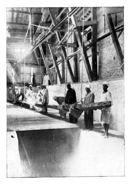
B.—Putting wooden boards (to cover the pit and serve as a ground) under the log after lifting it.
