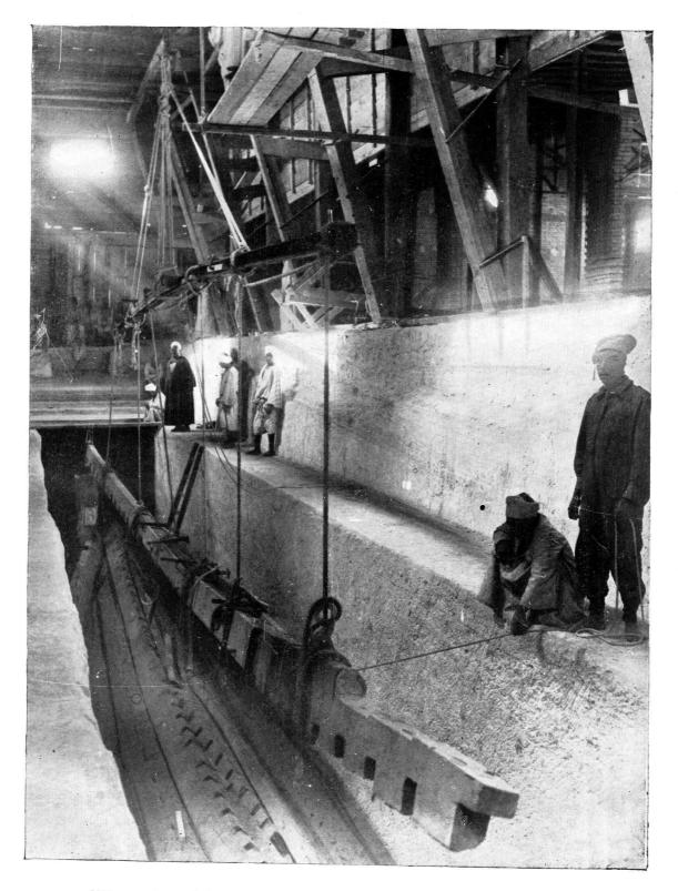
Lifting up the cracked piece with the fixed boards along the cracks. The crane, the beam and ropes can be clearly seen.
