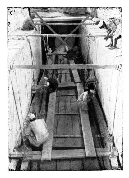
B.—Removing the skeleton of the scaffold and lifting the piece with ropes fixed at the pit-head.
